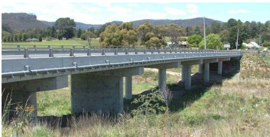
Lidsdale bridge in 2008 when the upper Sydney catchment was a lot drier than in earlier years.
